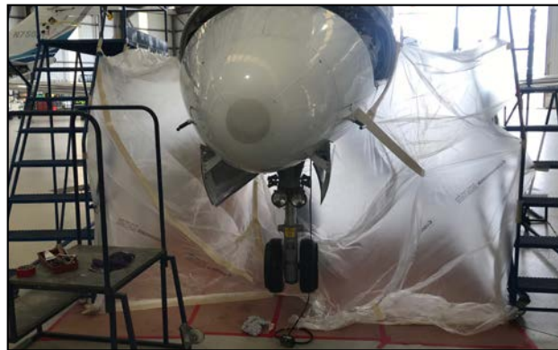
Build your tent with poly sheeting. Include inlets for make up air.
